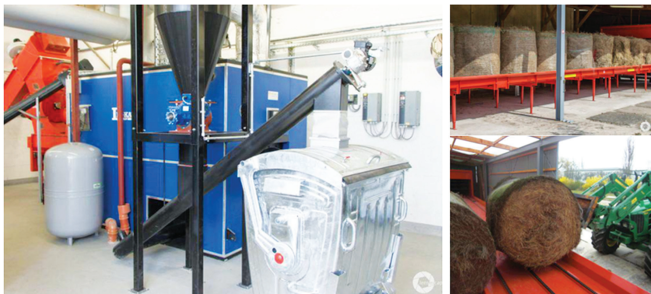
Fig. 2. 800 kW biomass boiler in Malchin for combustion of biomass from rewetted peatlands (Source: Agrotherm GmbH)
